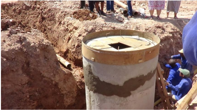
Construction of Manholes at Gibeon
